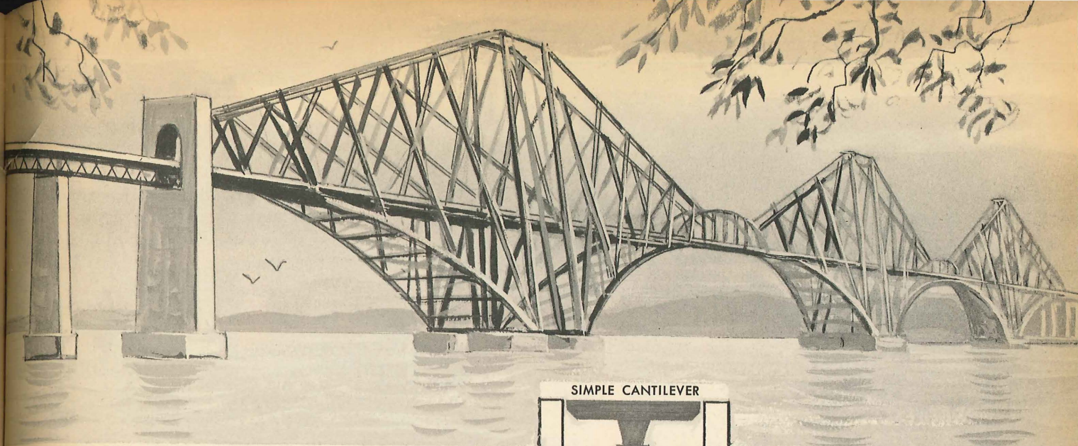
The first great cantilever bridge was over the Firth of Forth in Scotland.
